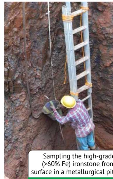
Sampling the high-grade (>60% Fe) ironstone from surface in a metallurgical pit.
